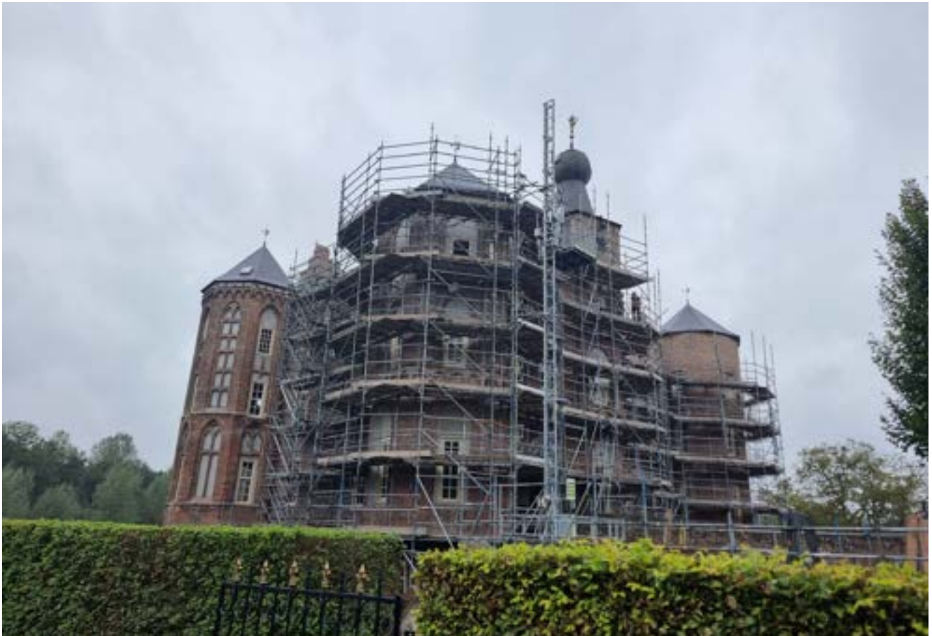
Foto 9 | Kasteel Croy in de steigers.
